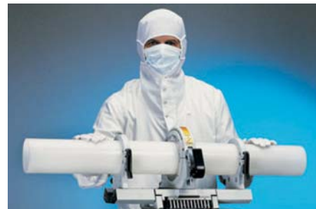
Joining ultra-high purity PVDF piping in a semiconductor plant
