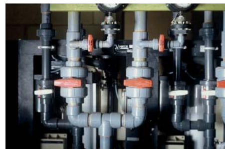
PVC and CPVC piping system in a chemical processing application
